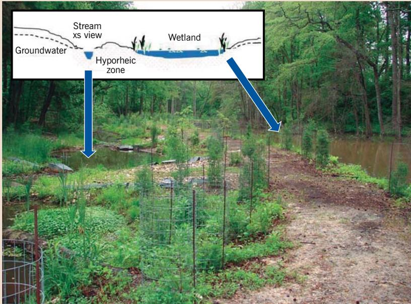
**Figure 11.9:** *Wilelinor is an ecologically engineered ecosystem combining both stream and wetland elements. The inset shows a cross-section schematic of the plan whereby the stream and wetland are hydrologically connected via overland flow during high discharge events and continuously via hyporheic flowpaths (i.e. below ground flow) through a porous sand berm*
